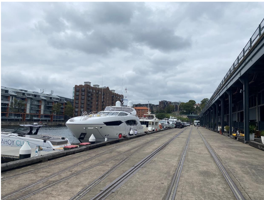
Figure 6: Eastern side of the wharf, looking towards Pirrama Road
