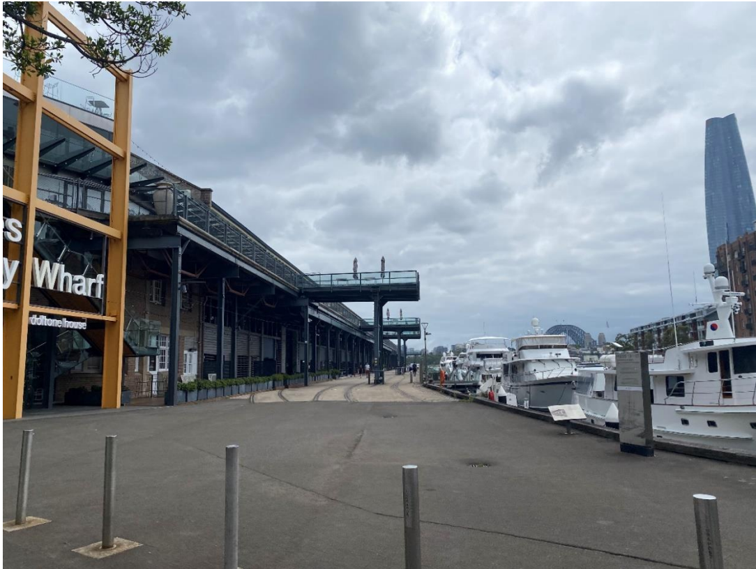
Figure 3: Site viewed from Pirrama Road, looking along the eastern side of the wharf
