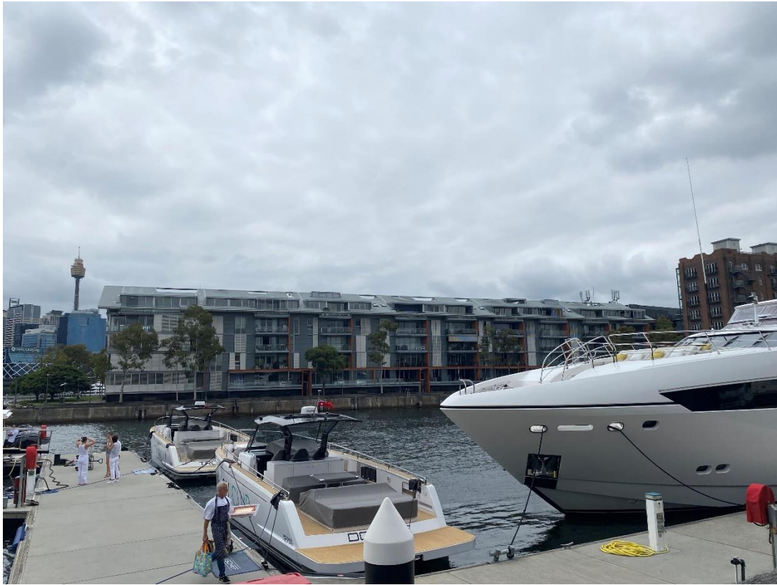
Figure 5: Eastern side of the wharf, looking towards the residential building at 3 Darling Island Road
