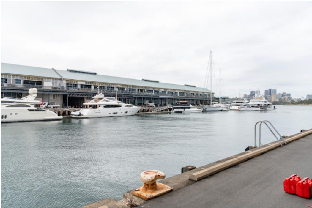
Figure 20: Before photo at Location 5 - Darling Island Walkway (south)
