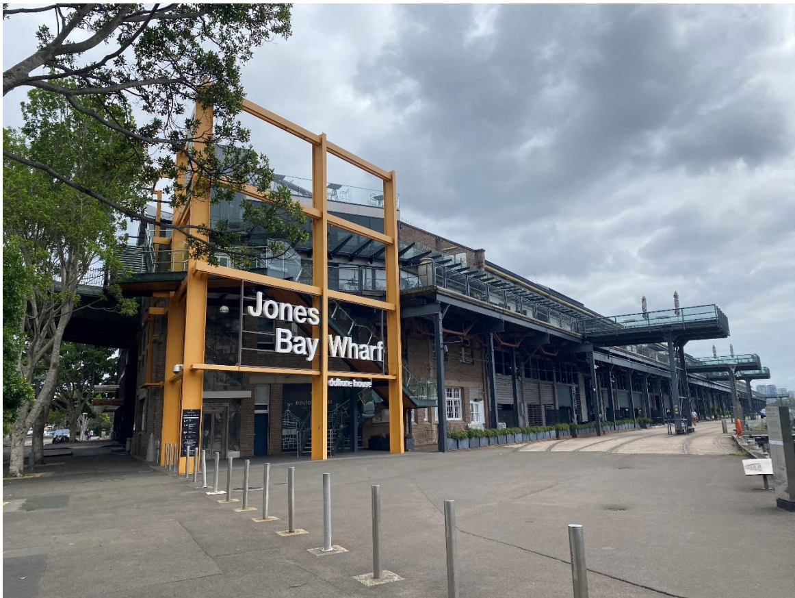
Figure 2: Site viewed from Pirrama Road, looking north
