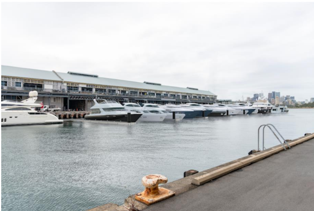
Figure 21: After photo at Location 5 - Darling Island Walkway (south)
